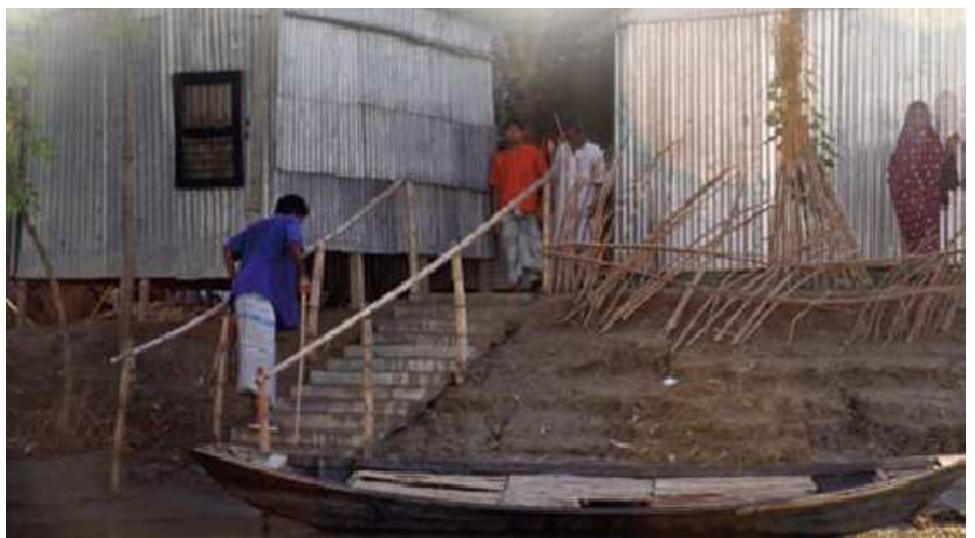
Accessible houses with stairs and handrails facilitating movement of persons with physical disabilities or with assistive devices.
